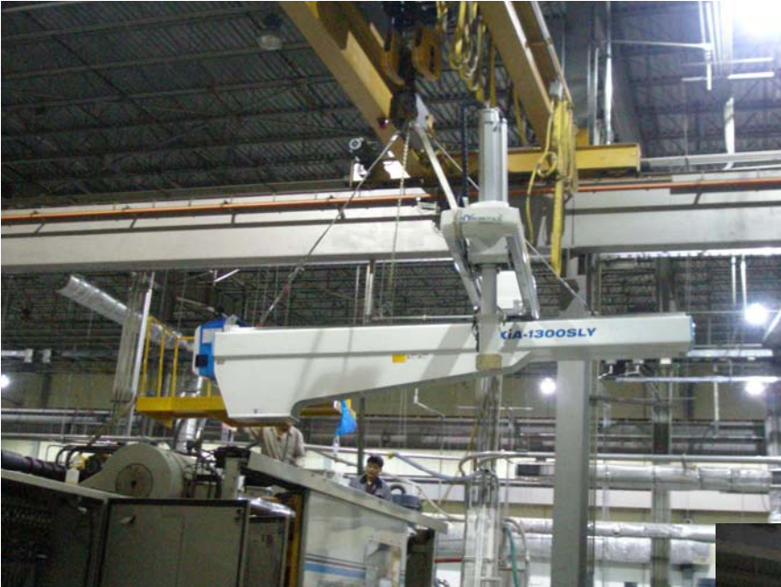
Robot Rigging for Installation : Secure and Safe Rigging
